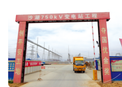
The service site of the 750kV Shahu Substation project in Ningxia
