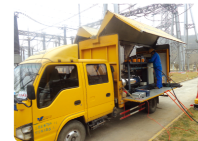
The service site of the 330kV Huangling Substation in Shaanxi
