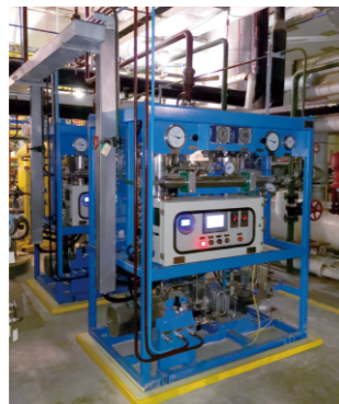
Shandong Huadian Tengzhou Power Plant
